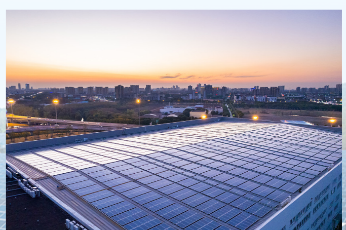
850KW photovoltaic power station project of a company in Guangzhou
