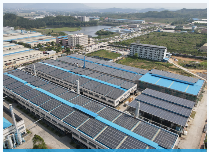
3MW photovoltaic power station project in a factory in Qingyuan
