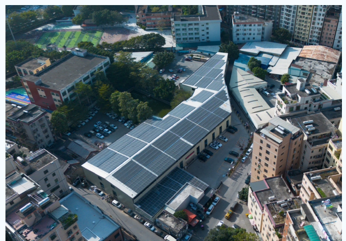
500KW photovoltaic power station project in a factory in Guangzhou
